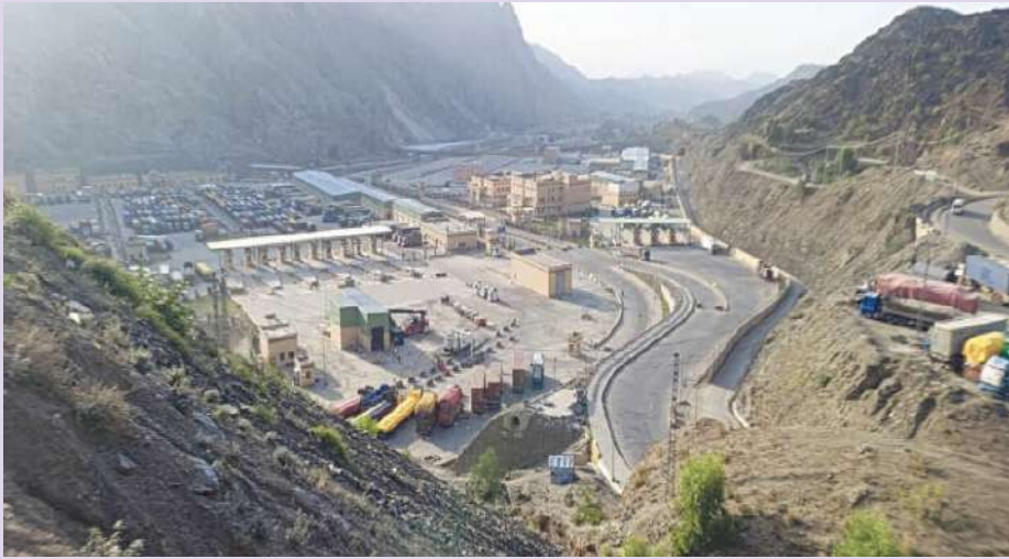
The newly-constructed Torkham customs terminal presents a deserted look.
