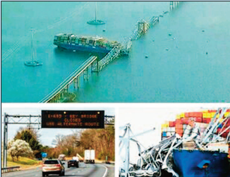
Bridge collapses in US on March 26, shows (Clockwise from top) an aerial view of the cargo vessel which crashed into the bridge; the steel frame of the bridge sits on top of the ship after it collapsed; and, a traffic warning sign is activated after the collision.
