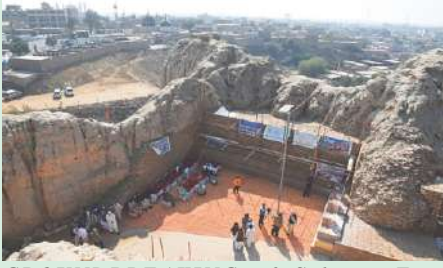
GROUNDBREAKING of Sehwan Fort preservation work being performed by Chief Minister Syed Murad Ali Shah along with several PPP ministers and lawmakers on Saturday 15 Jan.
