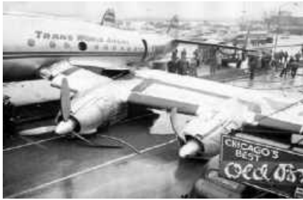
Technical Safety Issues from the Past
